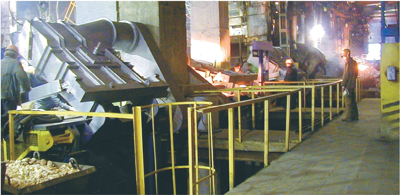
2x5 MW Converter with 3x8 ton Furnaces Triple Power System
